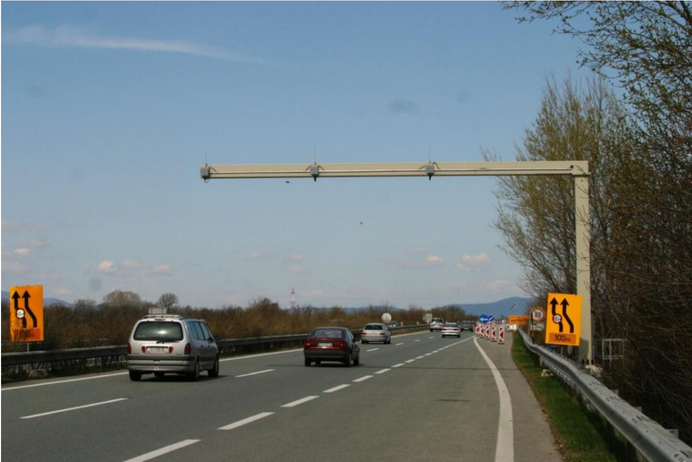
Heavy Goods Vehicle DSRC OBU detection point, Austria
