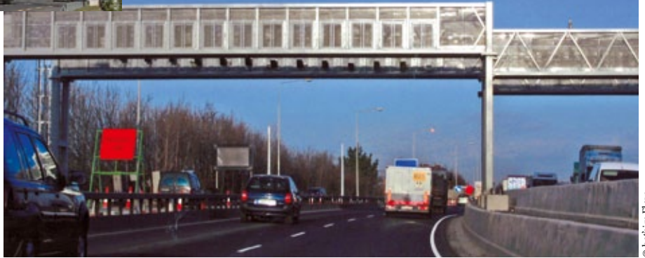
Multi-lane free flow charge point on the M50
